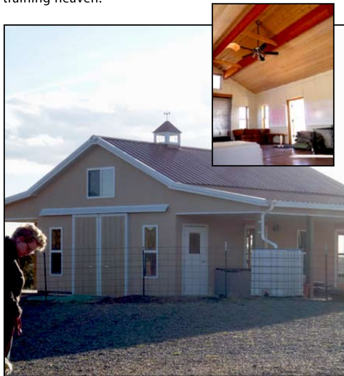
La Mariposa's Training Building for ADW. Inset shows inside the building.
